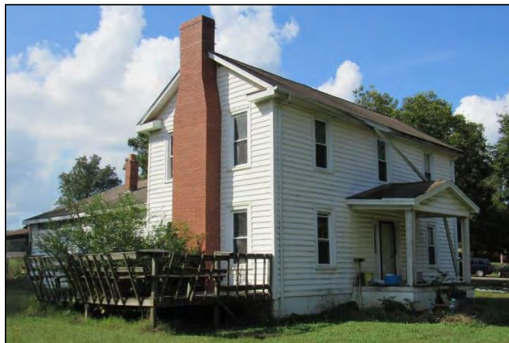
Photo 16: Southeast Oblique of J.B. Lutz House.
