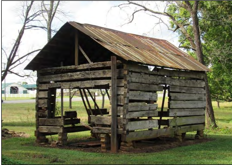
Photo 46: Log Kitchen, Northeast Oblique.
