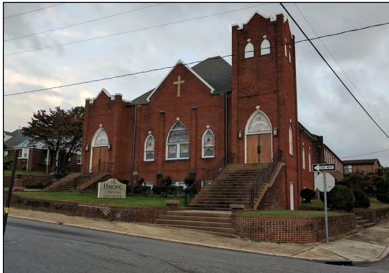
Photo 68: Northwest Oblique of the St. Paul's Lutheran Church (CT1366).
