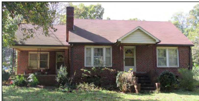
Photo 55: House at 2733 Startown Road, East Elevation.
