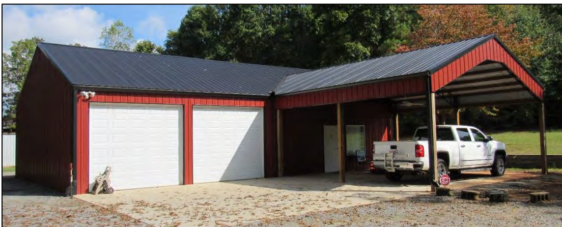
Photo 52: Workshop, Southwest Oblique.
