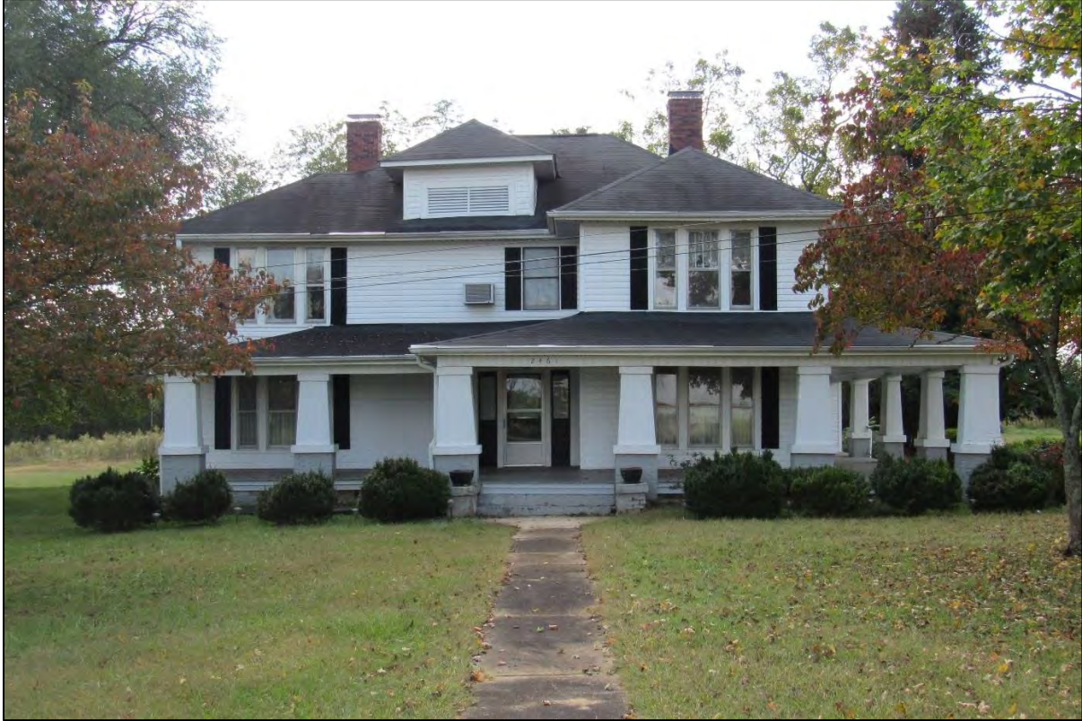
Photo 1: Northeast Elevation of the House at the W.R. Lutz Farmsite.
