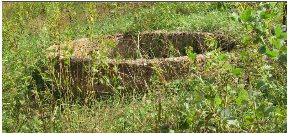
Photo 47: Silo Foundation, Looking North.
