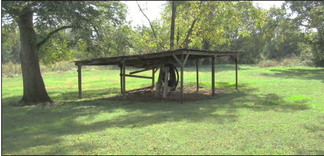
Photo 6: View of Open-Air Shed Looking Southeast.
