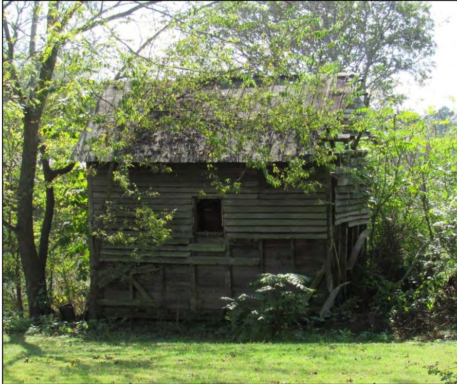
Photo 20: View of Domestic Outbuilding Looking South.
