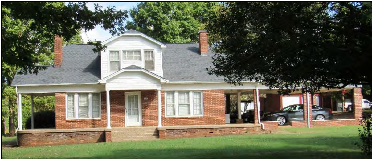
Photo 48: Single-Family Dwelling, South Elevation.
