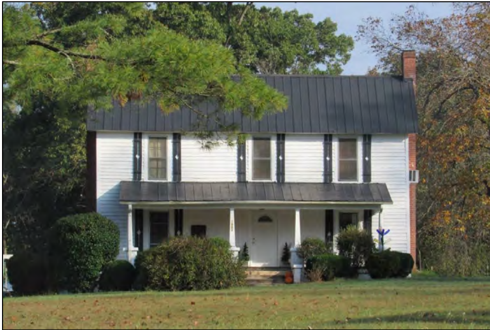
Photo 36: South Elevation of the House at 1882 Settlemyre Bridge Road (CT0564).
