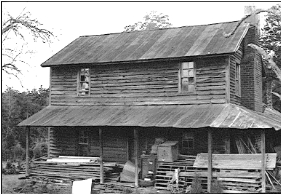
Photo 39: Photo of C.F. Bolick House from Previous Survey, North Oblique. 74
