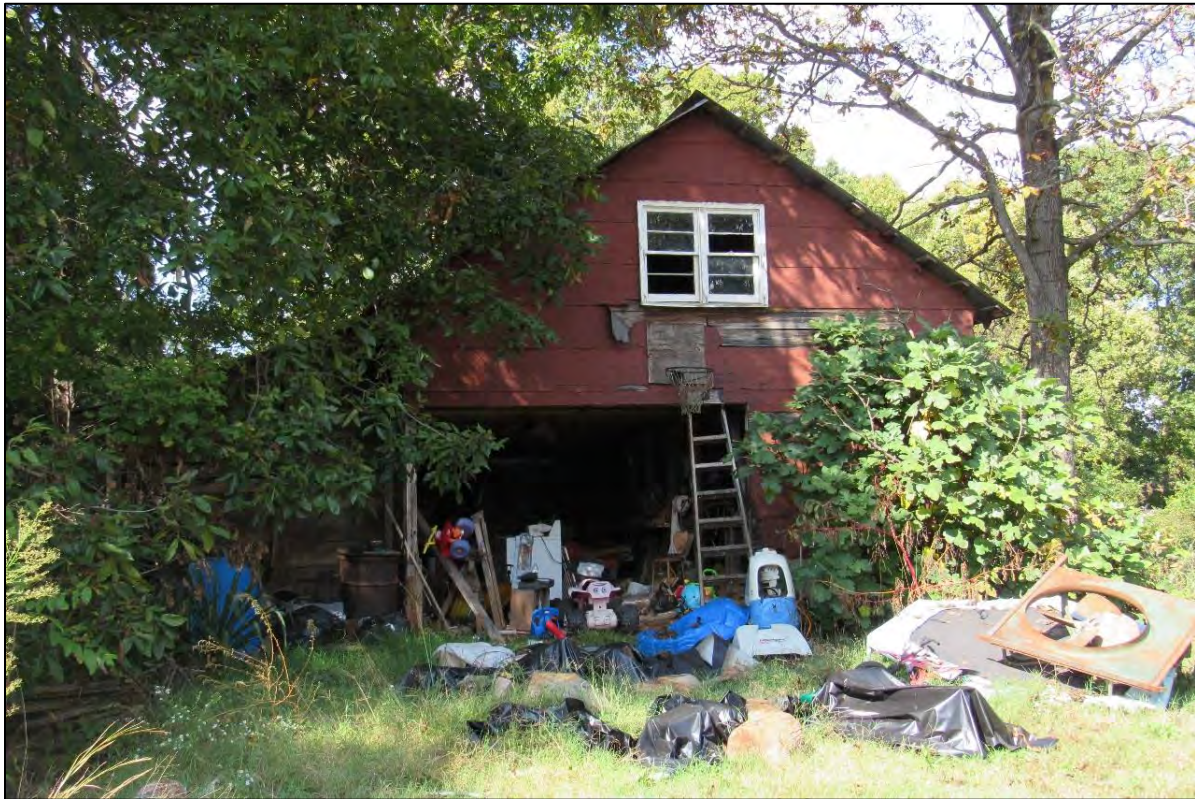
Photo 27: Southeast Elevation of Garage/ Workshop.
