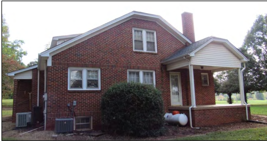
Photo 49: Single-Family Dwelling, West Elevation and Porch Detail.
