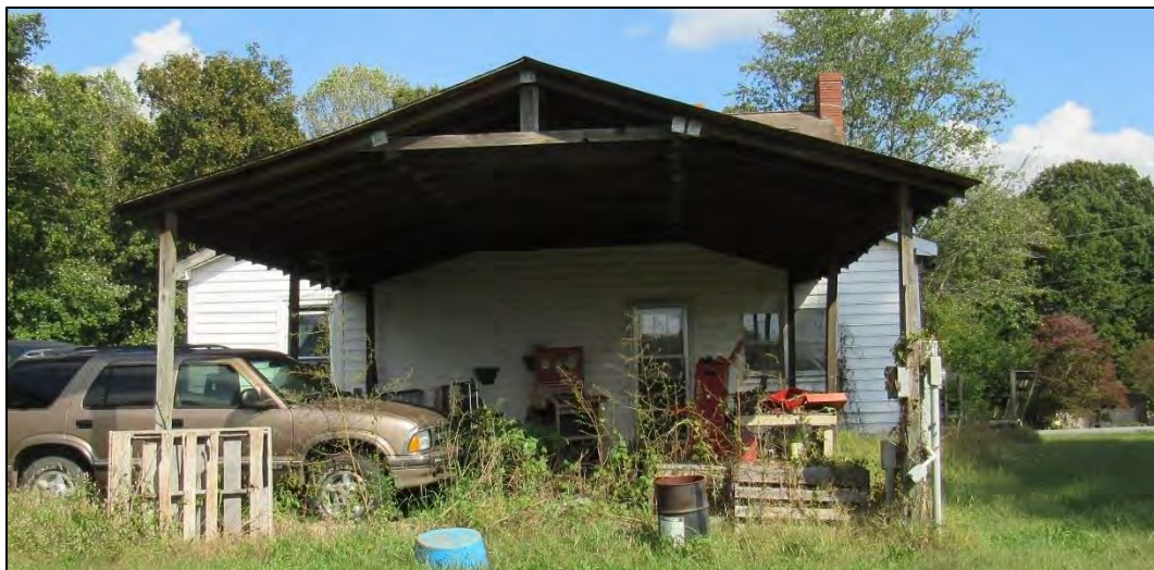
Photo 19: West Elevation of J.B. Lutz House.
