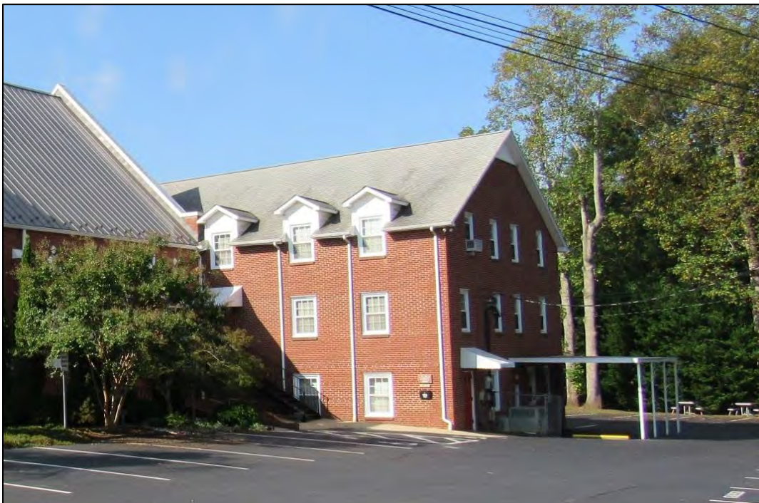
Photo 62: St. Paul Lutheran Church (CT1576), Addition Detail, Looking Southwest.
