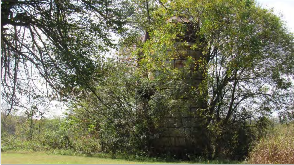
Photo 8: View of Silo Looking West.
