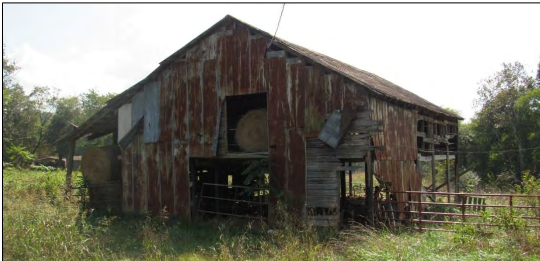
Photo 25: Northeast Elevation of Pole Barn.
