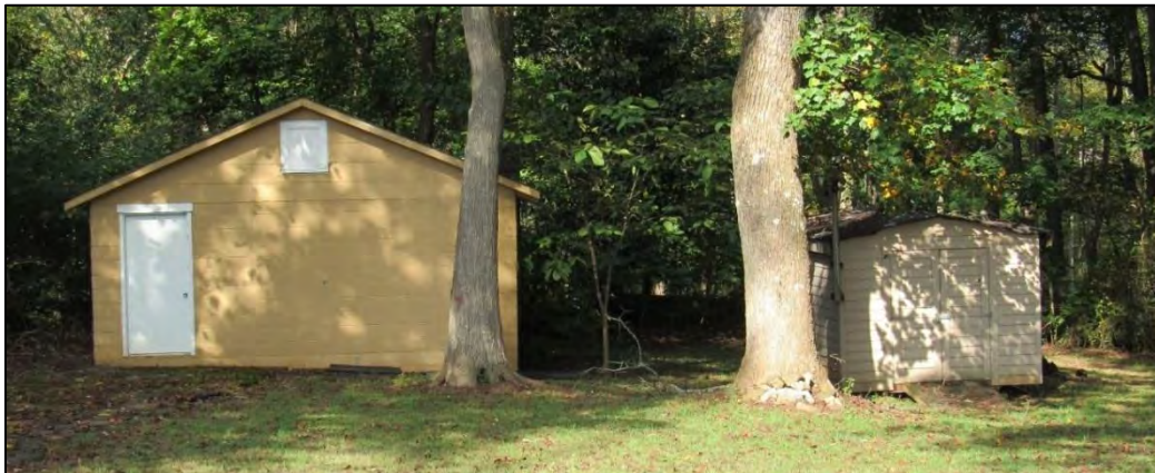
Photo 65: Storage Sheds, Looking West.
