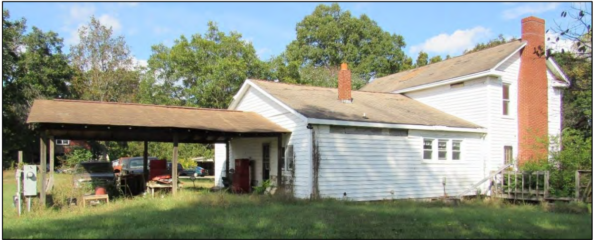
Photo 18: Rear Addition Detail of J.B. Lutz House, Southwest Oblique.
