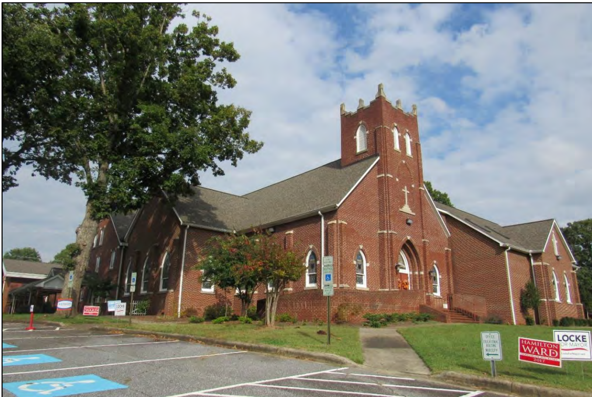
Photo 69: Southwest Oblique of the New Jerusalem Lutheran Church (CT1573).
