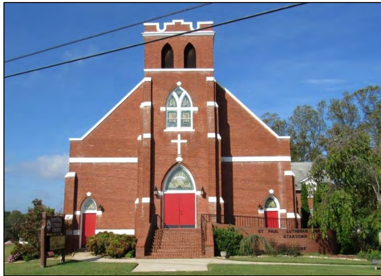
Photo 61: St. Paul Lutheran Church (CT1576), East Elevation.
