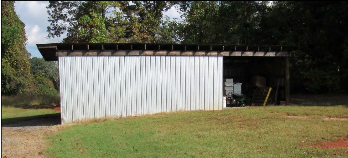
Photo 53: Machine Shed, South Elevation.
